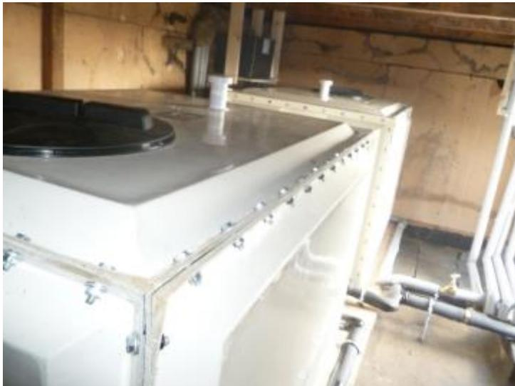
Each tank was cleaned and disinfected as it was put into service. Pipework in the flats below was checked at the end of each day to ensure that airlocks had not blocked supply as the tanks were refilled. Once the system was fully functional, pipework was insulated, tanks labelled and valves tagged.
