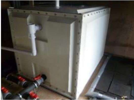
The existing tanks were, in turn, isolated and cut into sections with power saws. A new base of RSJs, treated against corrosion was installed and the GRP sections bolted together.
